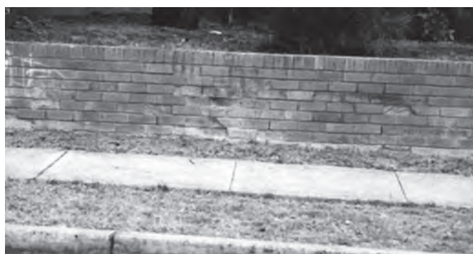
Bricks showing signs of salt and water . Source: DIPNR
