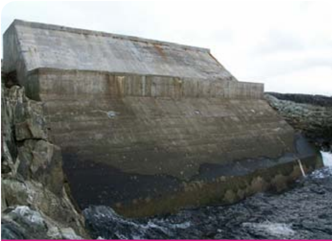
Wave energy power plant, Islay The LIMPET (Land Installed Marine Power Energy Transmitter) is the world's first commercial scale wave energy plant. It can supply up to 500kW and is connected to the national grid. Source: Claire Pegrum/Wikimedia Commons
