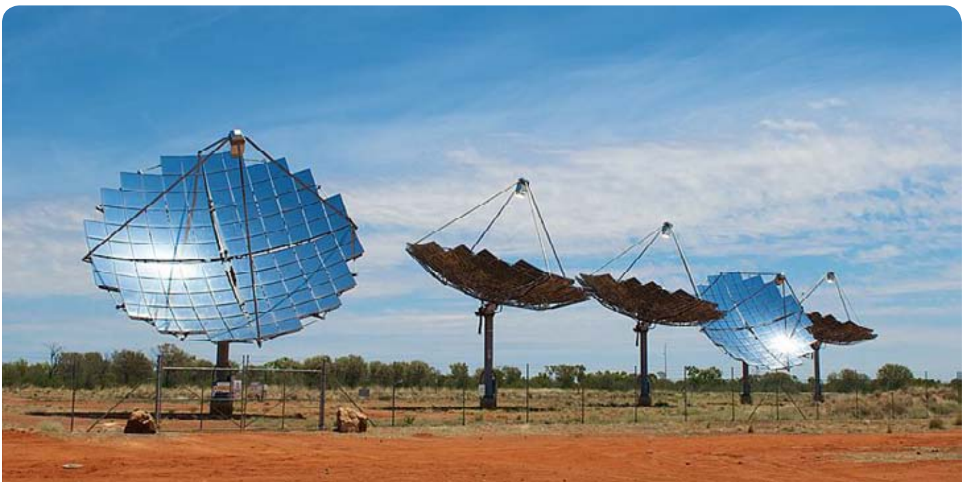
Windorah's Solar Farm dishes taken from the roadside (Diamantina Developmental Road) on a hot summer day. Source: Aaronazz/Wikimedia Commons
