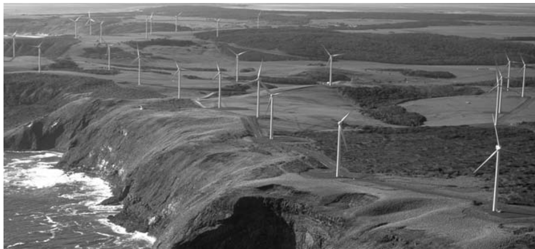
Woolnorth Wind Farm. Source: Hydro Tasmania
